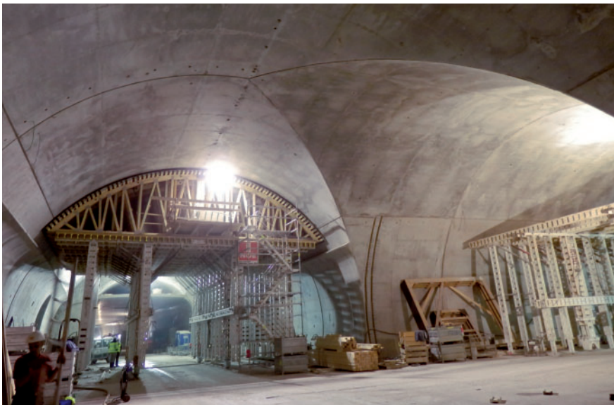
Finished ventilation gallery/tunnel tube intersection at emergency bay 2
