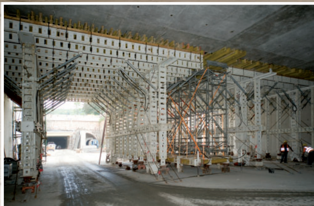
Left: Cut-and-cover tunnel construction east: the formwork carriage in the background is being prepared for the move from the south to the north tube Right: Cut-and-cover tunnel construction west: the NOEtec formwork carriages must allow site vehicles to pass through them to service the rest of the site. Formwork supported by loadbearing towers fills the gap in the area of the road alignment shift.
