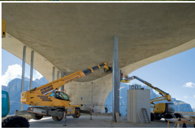
The ceiling soffit with the plaster-like finish of NOEplast texture Trier 3 ensures good room acoustics prevail in the hall. Approximately 400 m 2 of textured formliners were used in total. Uniform mat sizes provide a secondary pattern to the ceiling.
