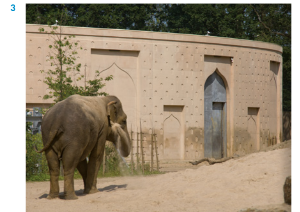
1 Flood protection wall in the Netherlands, individual pattern 2 MFA De Heerd in the Netherlands, customised anti-slip structure 3 Planckendaal Zoo in the Netherlands, individual pattern
