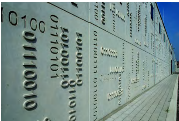
Data-Center Alpha-Cloud Mechelen, Belgien
